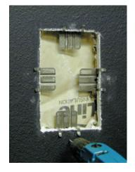
The Prest-on Insta-Backs fasteners make drywall repair quick and easy.
