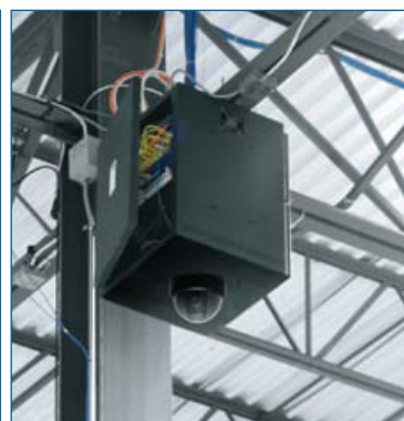
a typical warehouse IDF installation with optional dome camera mounted underneath
