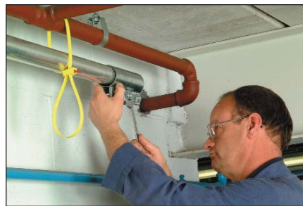
Suspended piping - SpeedyTie is ideal as a temporary support aid during the installation of gas, water, and air pipes.
