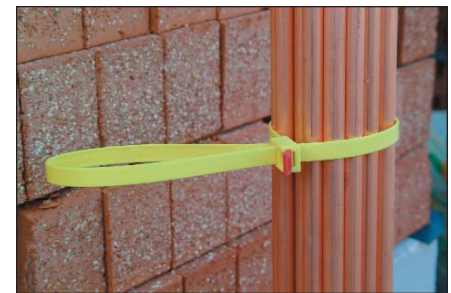
Site storage - bundling copper or plastic tubing together at the job site. Excess tail can be tucked away neatly for added safety.
