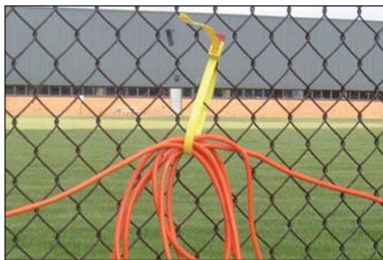
Temporarily attach extension cords or other cable to fencing.
