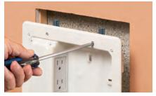
Tighten mounting wing screws to secure box to wall. As needed, attach box to block for added stability (see photo in 5 below).
