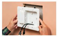
2 Wire receptacle. Install cover. Drop assembly and cable through the top hole, feeding it toward the bottom hole. Insert box in top hole, pulling cables for TV through opening in box.
