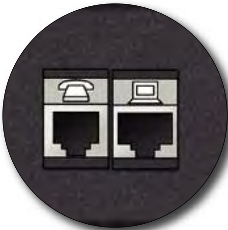
Telecom plate with RJ11 cat 3 phone and RJ45 cat 6 data.
