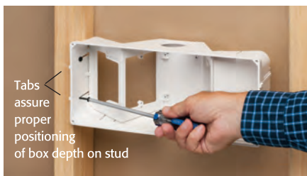
1 Attach box to stud through slotted holes.
