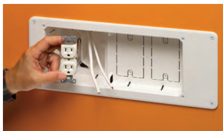
3 Install power and low voltage wiring devices.
