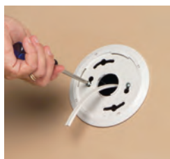
3 Install mounting plate per manufacturer's instructions
