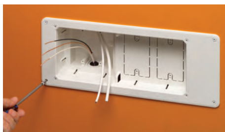
1 Install NM94 cable connector, and power and low voltage cables.
