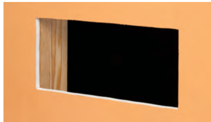
1 Cut hole next to stud (use enclosure, without trim plate, as a template). Pull wires. Insert box.
