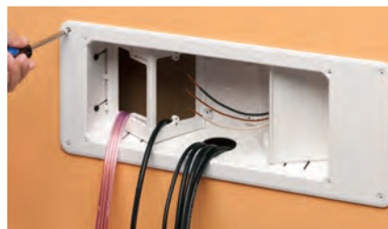
3 Install enclosure assembly to wall with outer screws.
